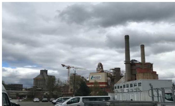
Project site of Lafarge Cement Plant
